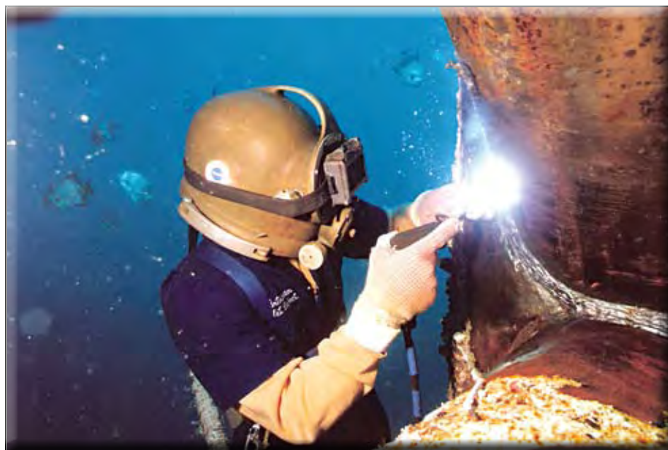
Innovative Welding Service owner Andrew Saltsman applies what he learned welding underwater then to his work on land today.
